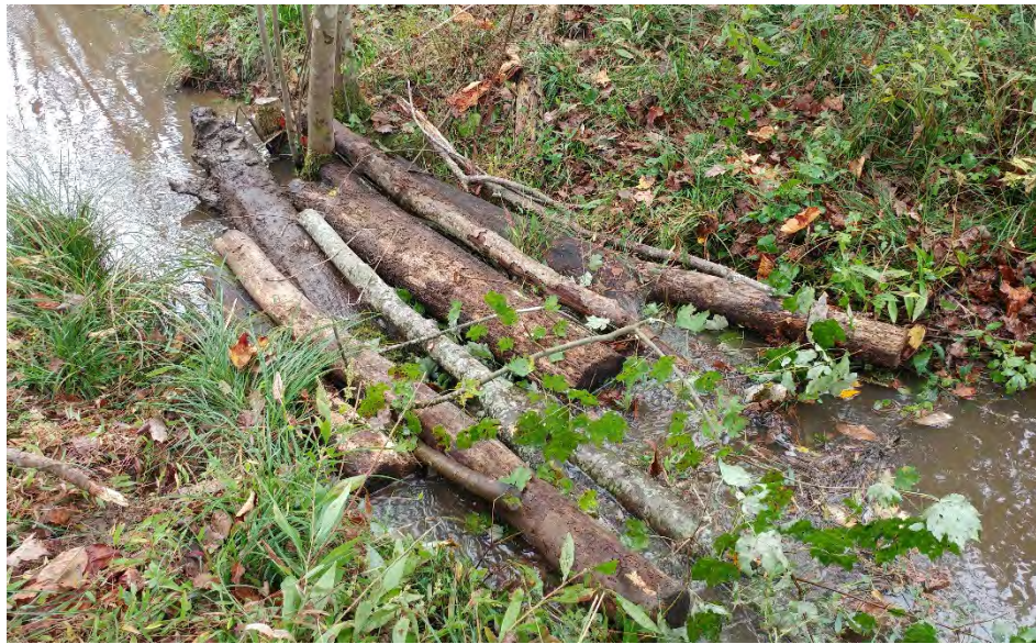
FIG. 3. The natural debris check dam installed in the stream and secured with rebar on October 13, 2017.
