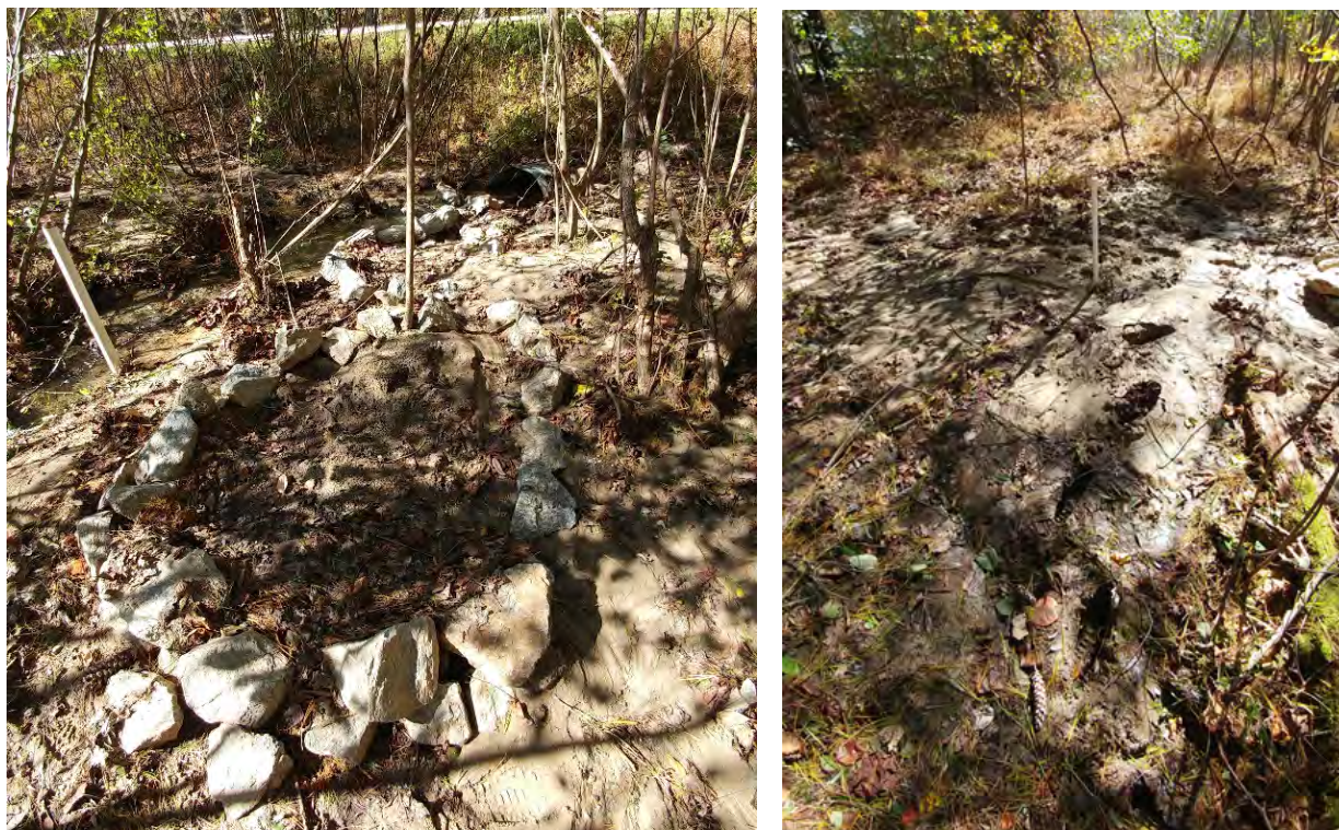
FIG. 12. (a) Left. The modified step-pools filled with sediment causing them to be ineffective at redirecting water to the east. (b) Right. The area to the east of the step-pools filled with sediment and visibly drier than when the step-pools are working.
