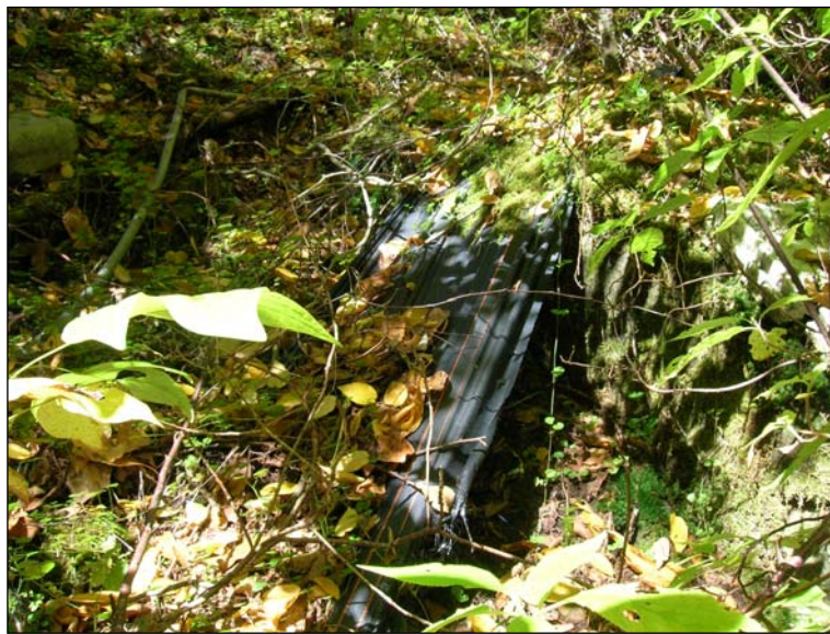
FIG. 9. Silt fence along stream bank of Tributary #1 which has been knocked over after the bank experienced mass wasting.
