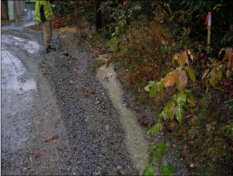
FIG. 8. Road adjacent from Tributary #1 which transports runoff sediment into the tributary.
